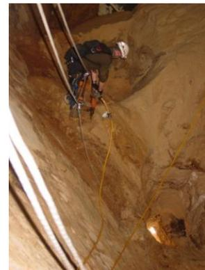
Figure 5: Cleaning Out of Sugar (Hygroscopic) Silo
