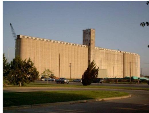
Figure 2: 1928 Burrus Elevator (slip form concrete steel reinforced) in Lubbock, TX just before demolition in 2004 contains 123 silos.
