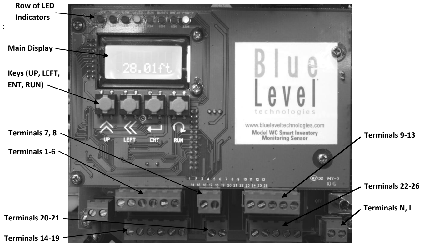
Figure 11: Main PCB with LCD display, configuration keys & terminal connections
